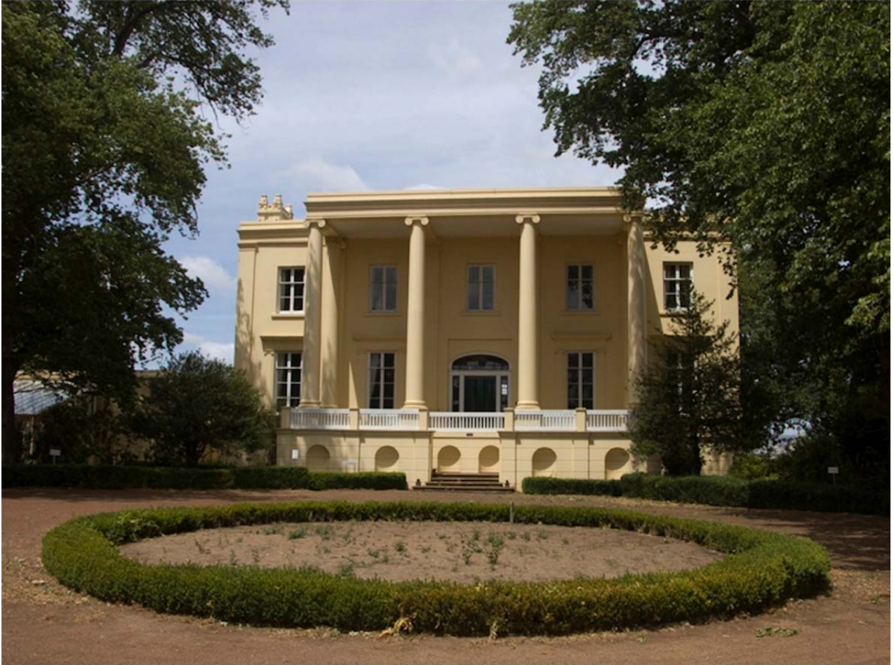
Clarendon House, Evandale prior to installation
