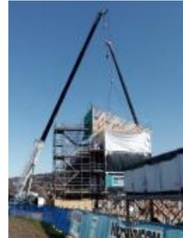
Figure 11: Line of modules with prefabricated roof units.
