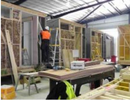
Figure 8: Modules under construction in the prefabrication factory.
