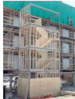
Figure 13: Prefabricated CLT stairs.
