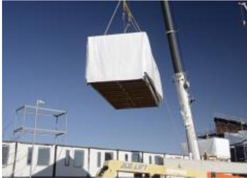
Figure 10: Modules being lifted into place.
