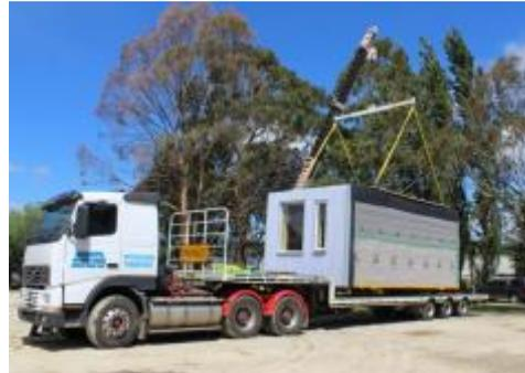
Figure 7: Wrapped and clad prototype lifted off after road testing.
