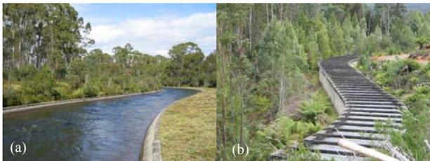
Figure 1. Tarraleah No.1 Canal (a) Trapezoidal in-ground canal section. (b) Rectangular above-ground flume section.
